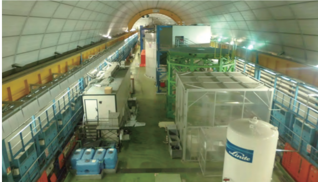
Fig.1 Underground laboratory of the Gran Sasso National Laboratory (LNGS), Italy
